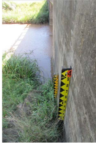
Figure 6.16: Gauging weir on the upstream side of the road bridge.
