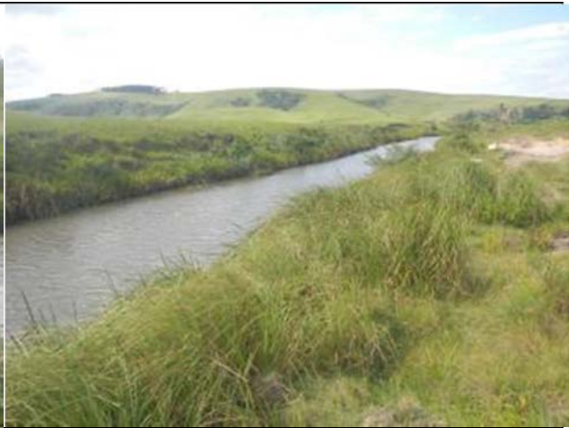
Figure 6.54 Downstream view of pipeline crossing
