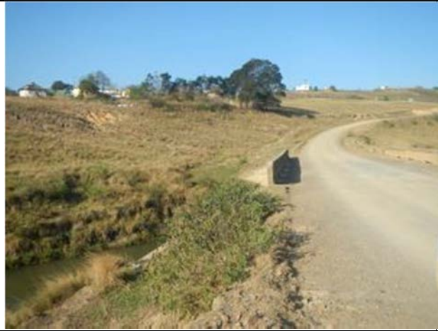
Figure 6.30. View of the river bank downstream of the road bridge.
