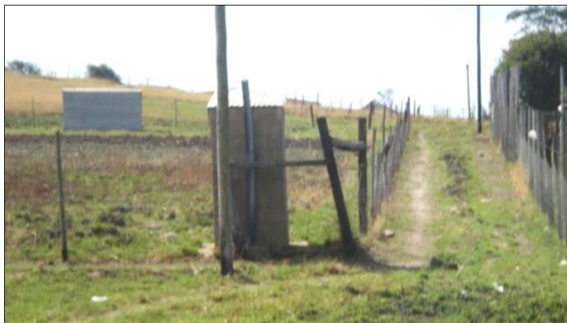
Figure 4.15: Ventilated pit toilet in the project area
