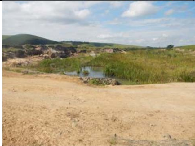
Figure 6.50 Upstream view of pipeline crossing
