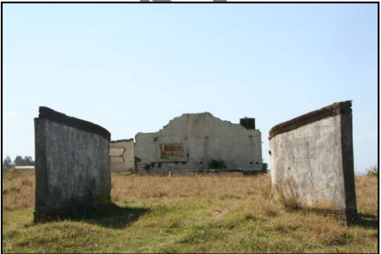
FIG.71: BUILDING AT LSS065
