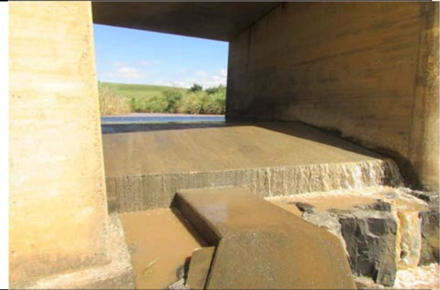
Figure 6.14 Existing abstraction weir.
