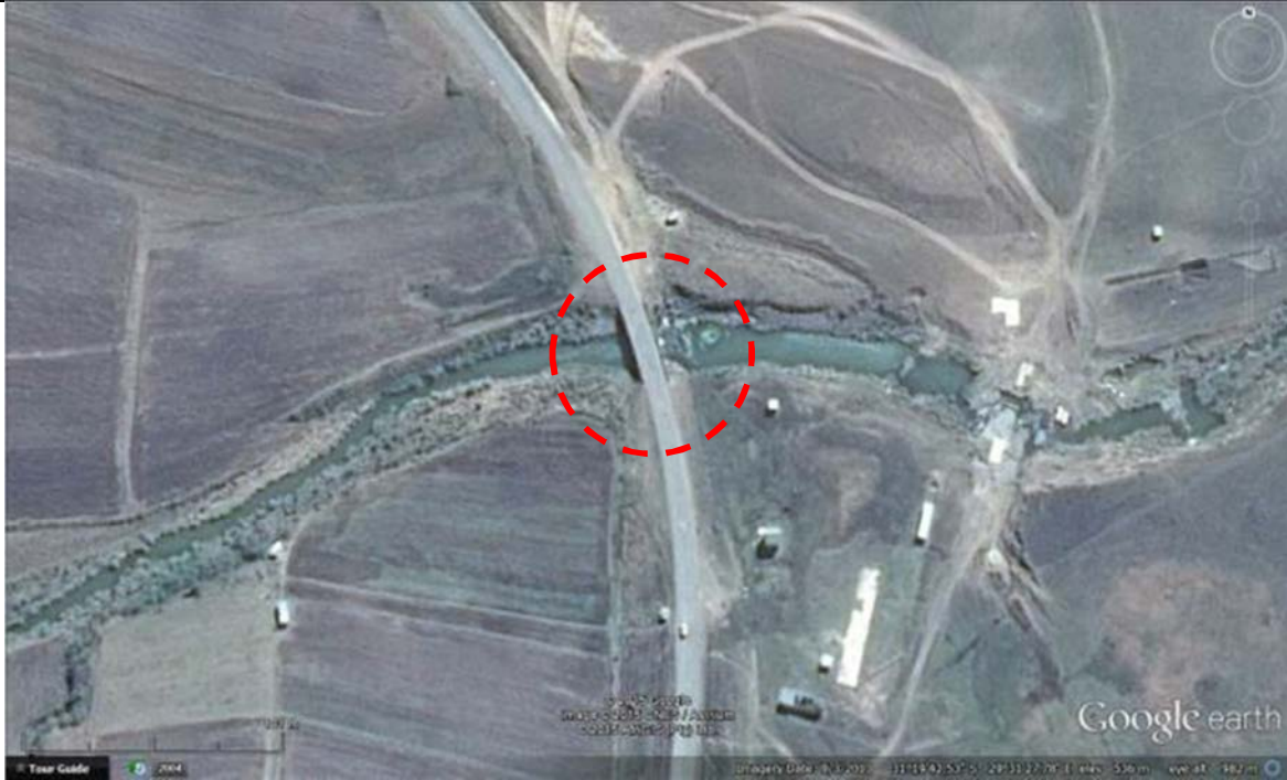
Figure 6.12. Aerial view of the abstraction weir site.
