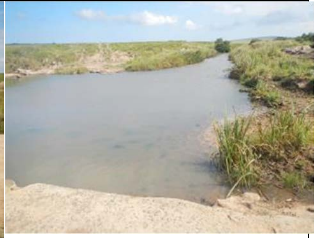
Figure 6.51 Downstream view of pipeline crossing
