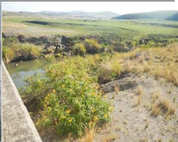
Figure 6.28. Downstream view of the Mzintlava River at the bridge.
