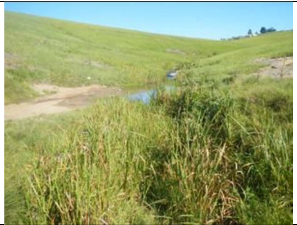
Figure 6.45 Upstream view of pipeline crossing
