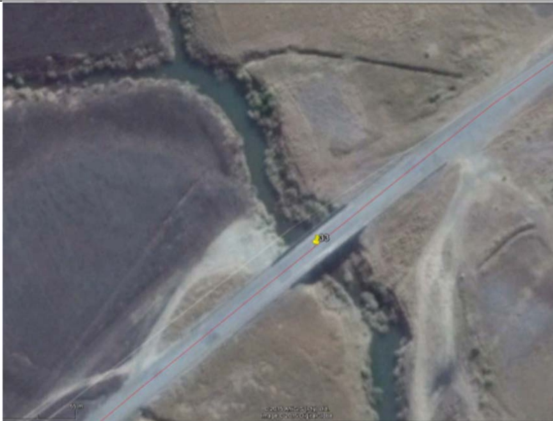
Figure 6.26. Aerial image of the pipeline crossing site
