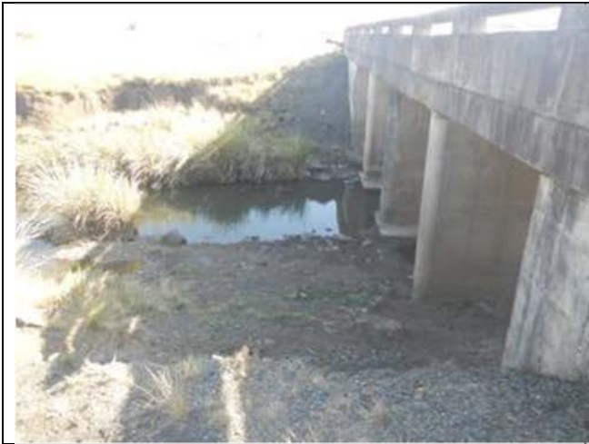
Figure 6.27 Upstream view of the Mzintlava River at the bridge.
