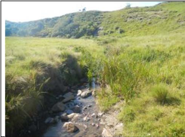
Figure 6.44 Downstream view of pipeline crossing
