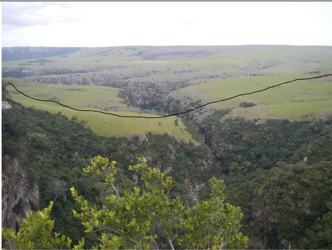
Figure 6.56. View of pipeline crossing
