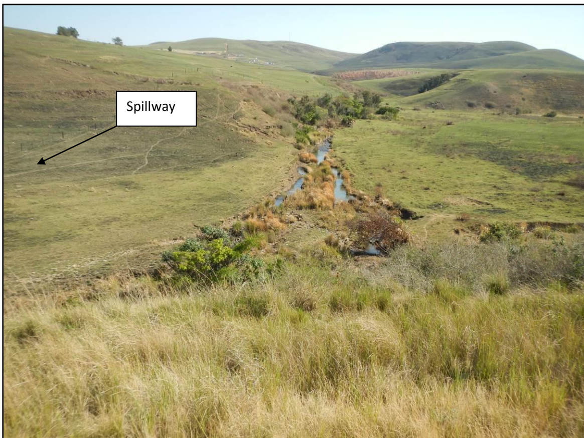
Figure 7.10 Spill way of Zalu Dam underlain by Eccca Group Shales (GPS: 31° 18' 43.5"S 29° 28' 30.00"E)
