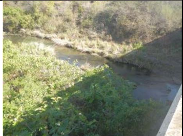
Figure 6.25: A view of the Mntafufu River upstream of the bridge. The banks are relatively shallow, with evidence of bank erosion present.
